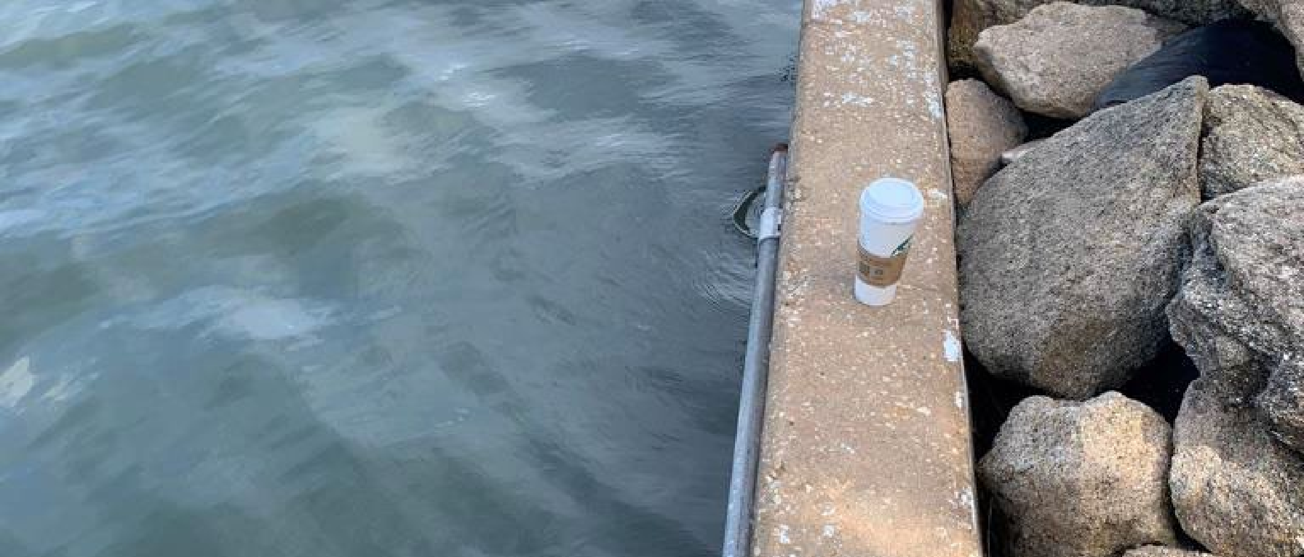
Cape Canaveral, Center St. Outfall (September 2021)
