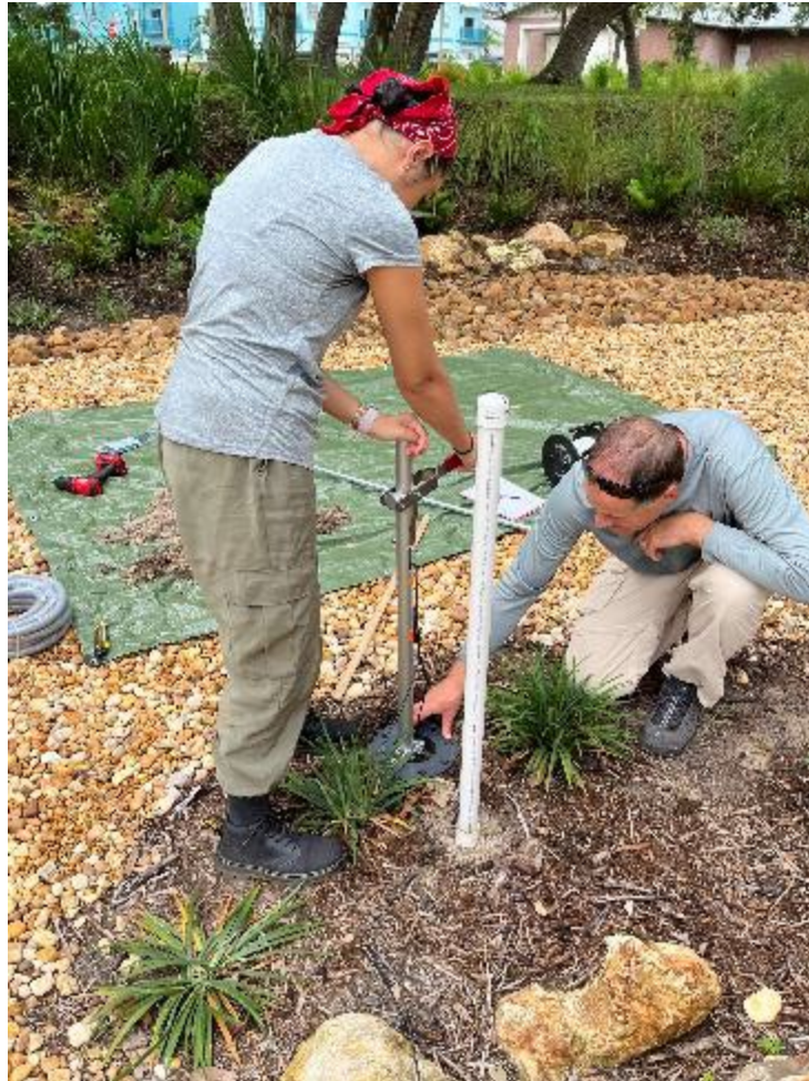
Figure 1: Soil sensor installs at Well 1
